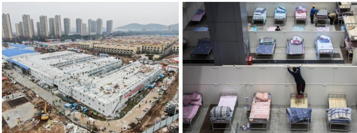
Left: An aerial photo shows the Huoshenshan Hospital in Wuhan, a makeshift hospital built in 10 days to house people infected with coronavirus. Right: Workers prepare beds at Wuhan International Conference and Exhibition Center. PHOTOGRAPH BY GETTY IMAGES
